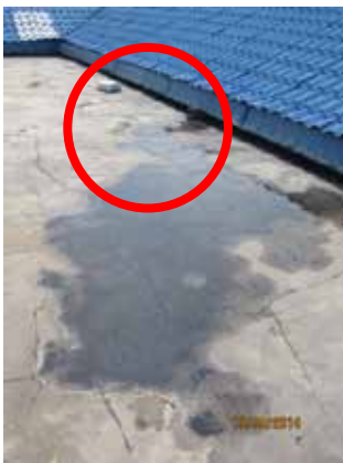
Figure 8: Condition of flat roof surface near RWDP 6 showing the existence of water ponding
