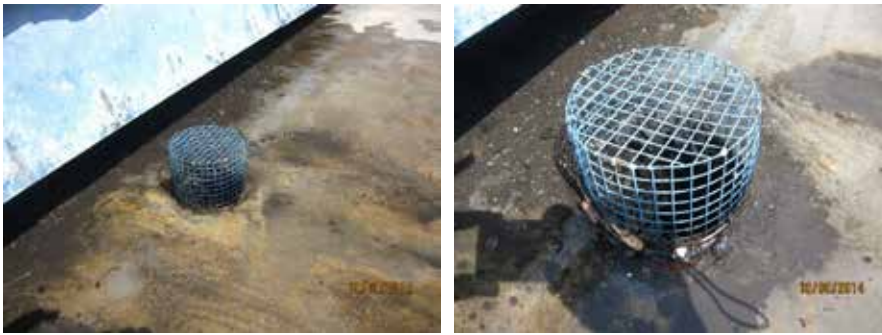
Figure 16: Efficient flow of water after cleaning the dirt around RWDP 2
