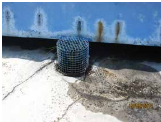
Figure 8: Condition of flat roof surface near RWDP 6 showing the existence of water ponding
