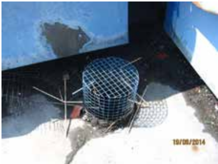
Figure 6: Condition of RWDP 4
