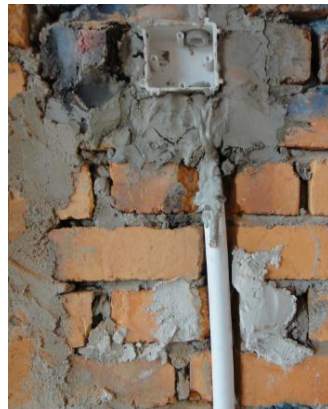
Hacking of bricks to embed M&E
