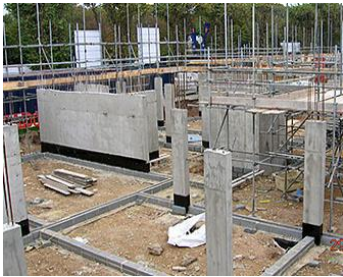
Slabs & walls are formed separately
