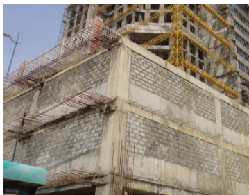
Costly & timing consuming brick laying & plastering (3-6 months)
