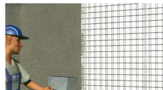
Spraying of the coating layer on the panel by using the plaster sprayer.
