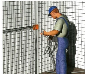
Spraying of the coating layer on the panel by using the plaster sprayer.
