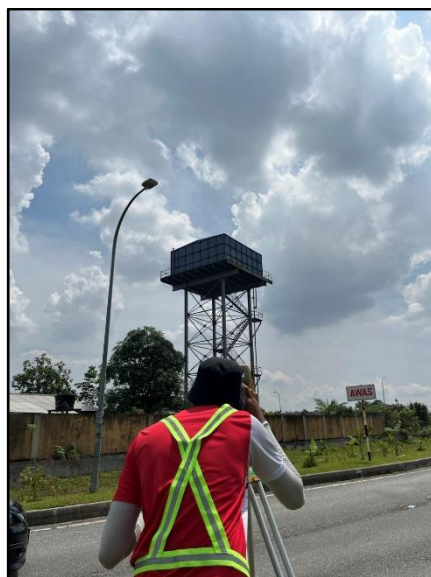
Figure 4: Transferring Coordinates to water tank structure
