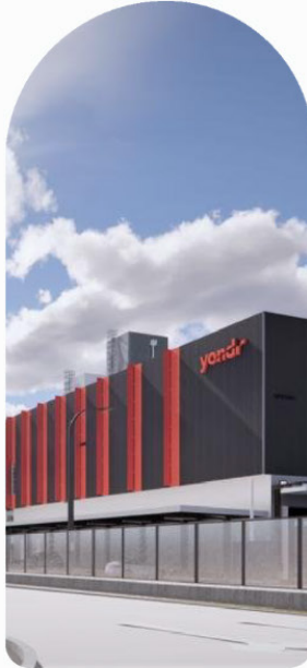
JHBX1 Data Center
