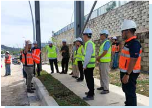
Site visit to Elmina Ridge 1
